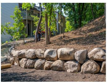
The crew spent a week rebuilding the large retaining wall behind unit #61, replacing one of the last pressure-treated lumber retaining walls left in the Association. It was a big project, involving removal of the old wall's timbers, and placement of many heavy boulders to create a much-more-permanent retaining wall that should last many decades.
