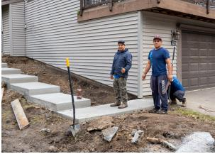
In early September the crew completed rebuilding the sidewalk behind units #226-#229 including steps on both ends of the building. The Association is slowly, one-by-one, replacing all steps and sidewalks in the Association with rebarred concrete designed to last for years.
